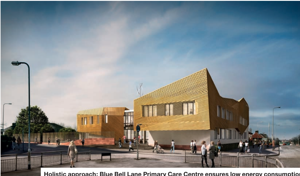
Holistic approach: Blue Bell Lane Primary Care Centre ensures low energy consumption
